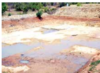
Digging new pond for rain water conservation
